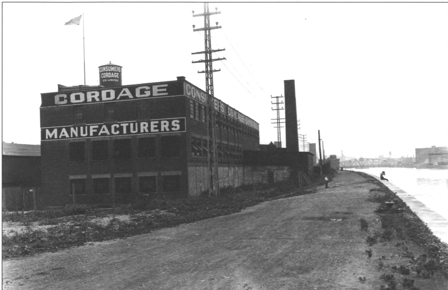
L'usine Cordage Manufacturers, 1942. Archives nationales du Canada (PA119176). Cordage Manufacturers factory, 1942. National Archives of Canada (PA119176).
