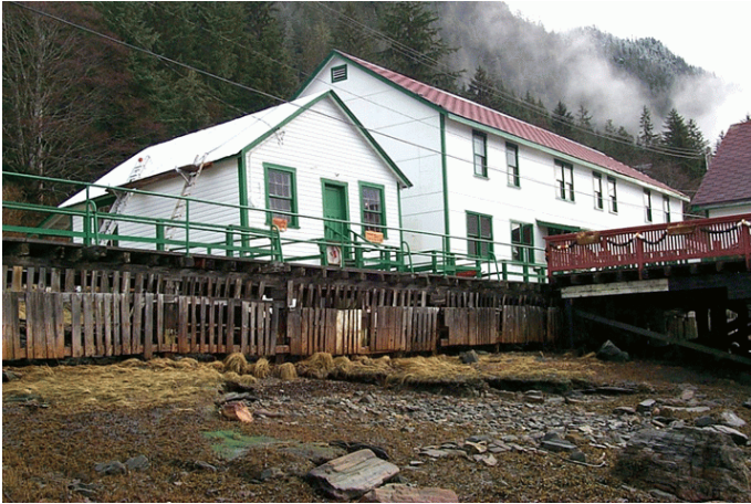
Photo 5 Upper intertidal habitat. Note wooden skirt on boardwalk. L to R Lineman's House, Two Storey Bunkhouse (Bed & Breakfast), portion of Mess Hall. Intertidal type 2 present here. 21 February 2000
