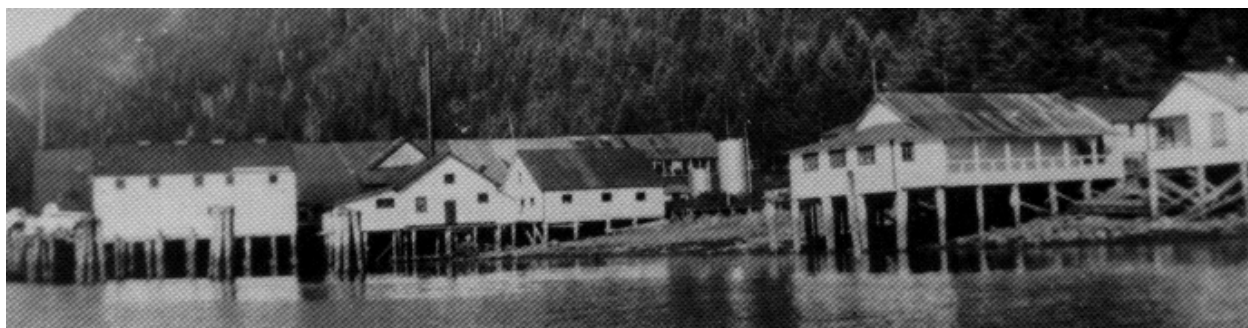
Figure 3: North Pacific Cannery during the 1940s. The buildings in front of the main cannery are the ice house and the old cold storage and reduction plants. These were replaced by the larger reduction plant. At right is the store with the office in the extension over the water. (NP photo, Ross Collection.)
