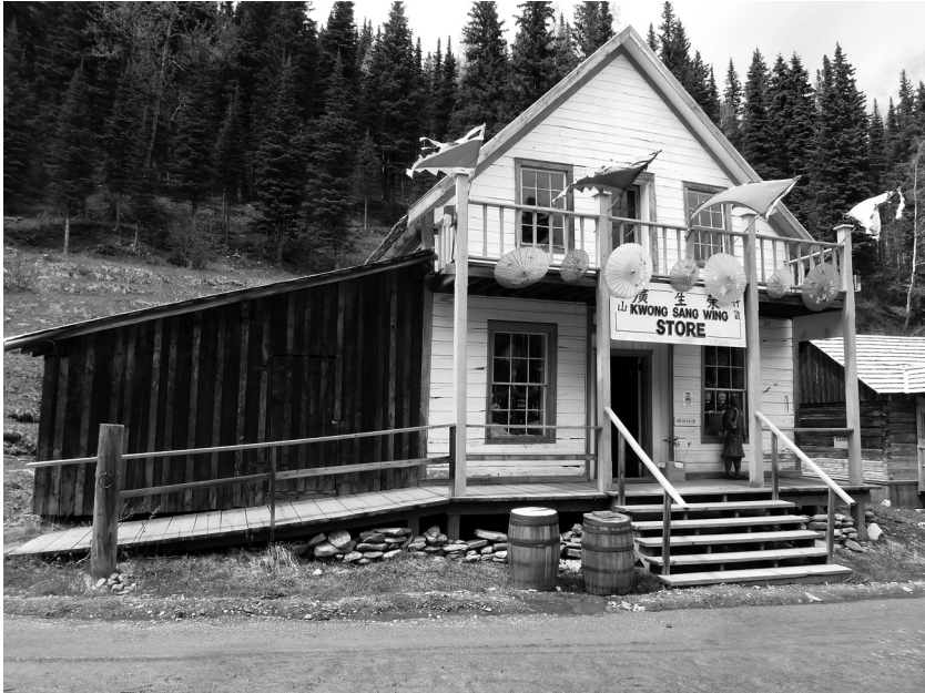
Figure 2. Kwong Sang Wing Building, Barkerville. Photo by author.
