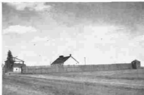
View of Stockade showing Main Gate and Bastion, Fort Battleford National Historic Park.
