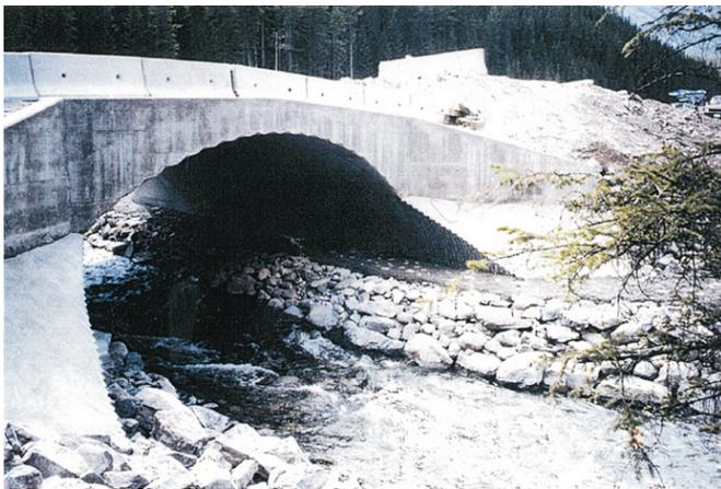
Fig. 9. Wildlife underpass 4 x 7 m culvert.
