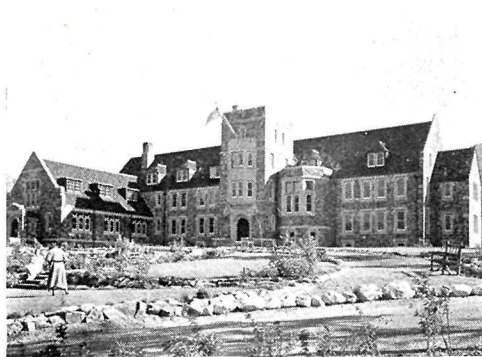
Banff Park Administration Building.
