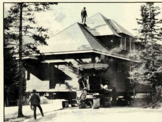
Even the train station was hoisted from its foundations and moved out
