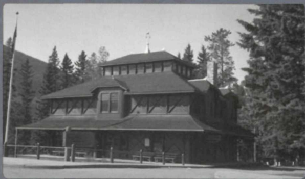
▲ Banff Park Museum, a typical example of the Rocky Mountain Architectural Style V488/327 (1)
