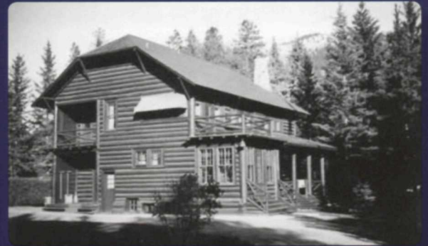
▲ The Park Superintendent's residence on Buffalo Street in 1937, Block B Lot 3-5
