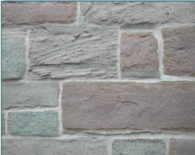
**Figure 8. Stone blocks made of Sillery sandstone**
