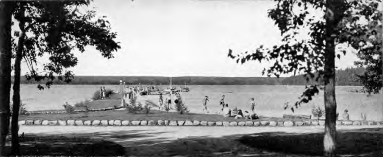
The Breakwater and Dock at Wasagaming
