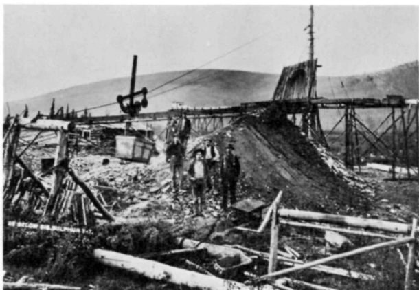
Shaft and Drift work on Sulphur Creek.
