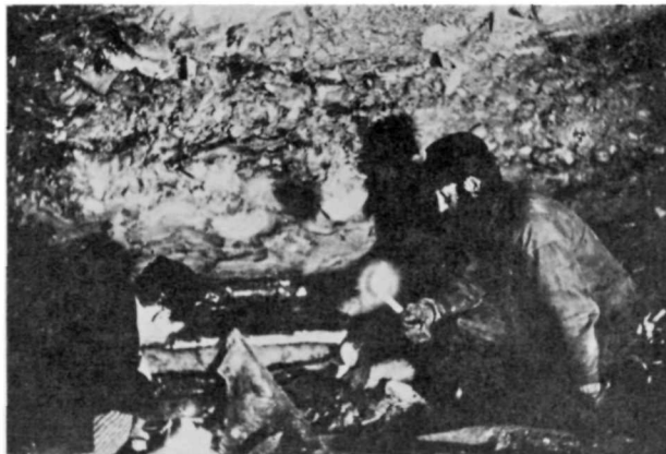
Thawing with wood and by steam. The wood was so cold that the miners set their fires with candles instead of matches.
