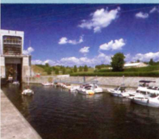
The lock's "guillotine" gate
